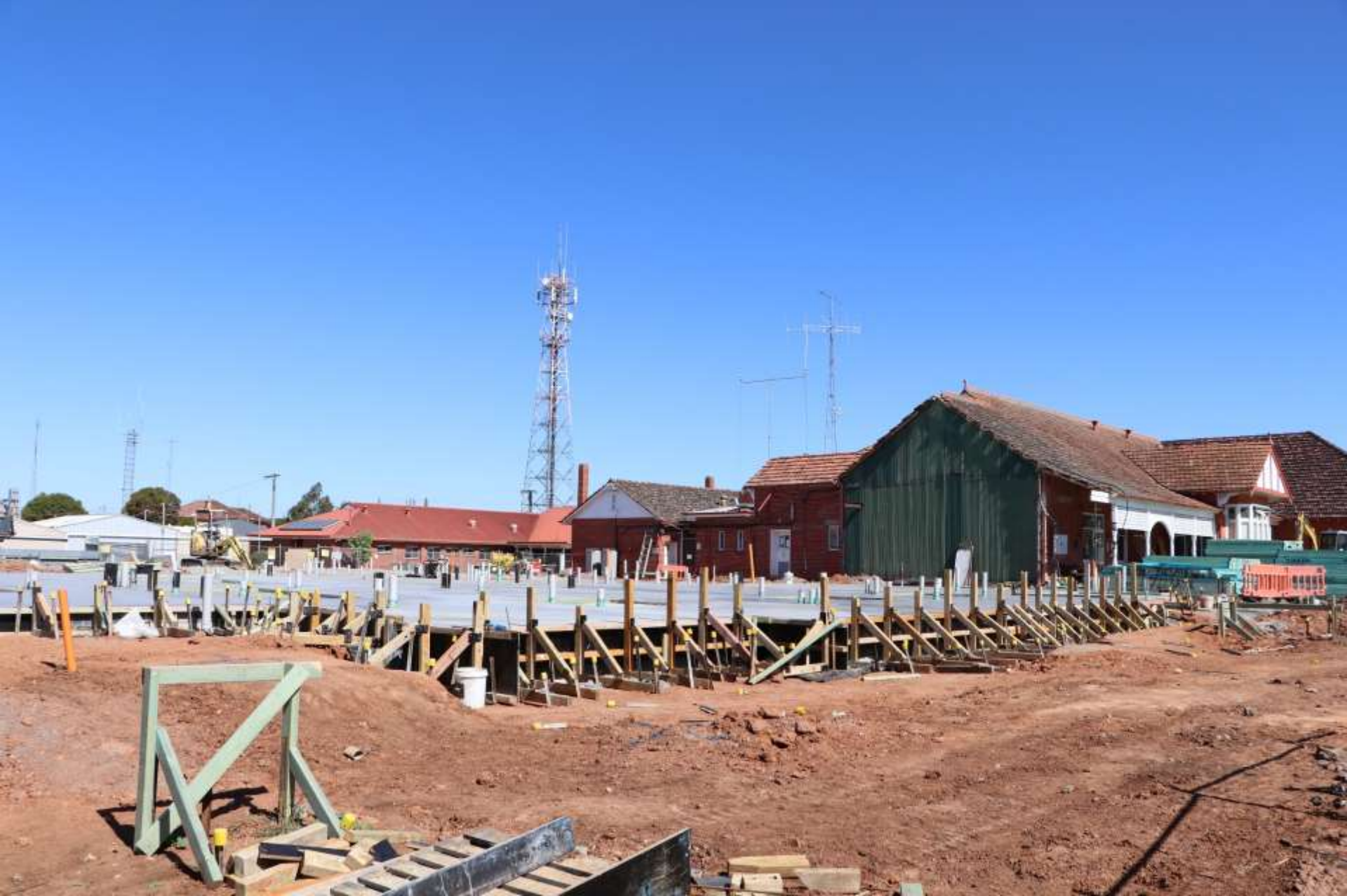
EWHS Birchip Campus – Hospital Foundations
