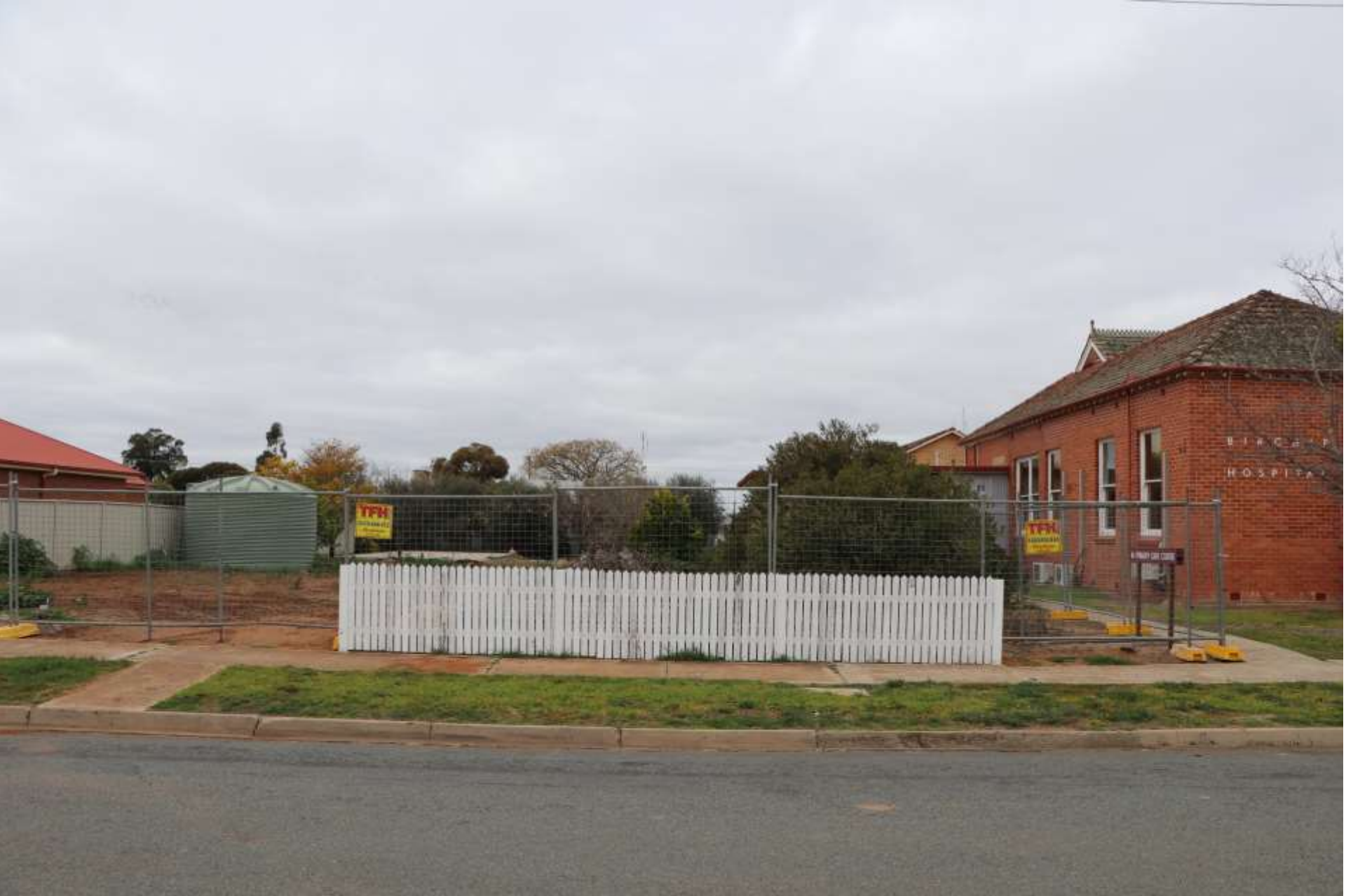
EWHS Birchip Campus – After Demolition
