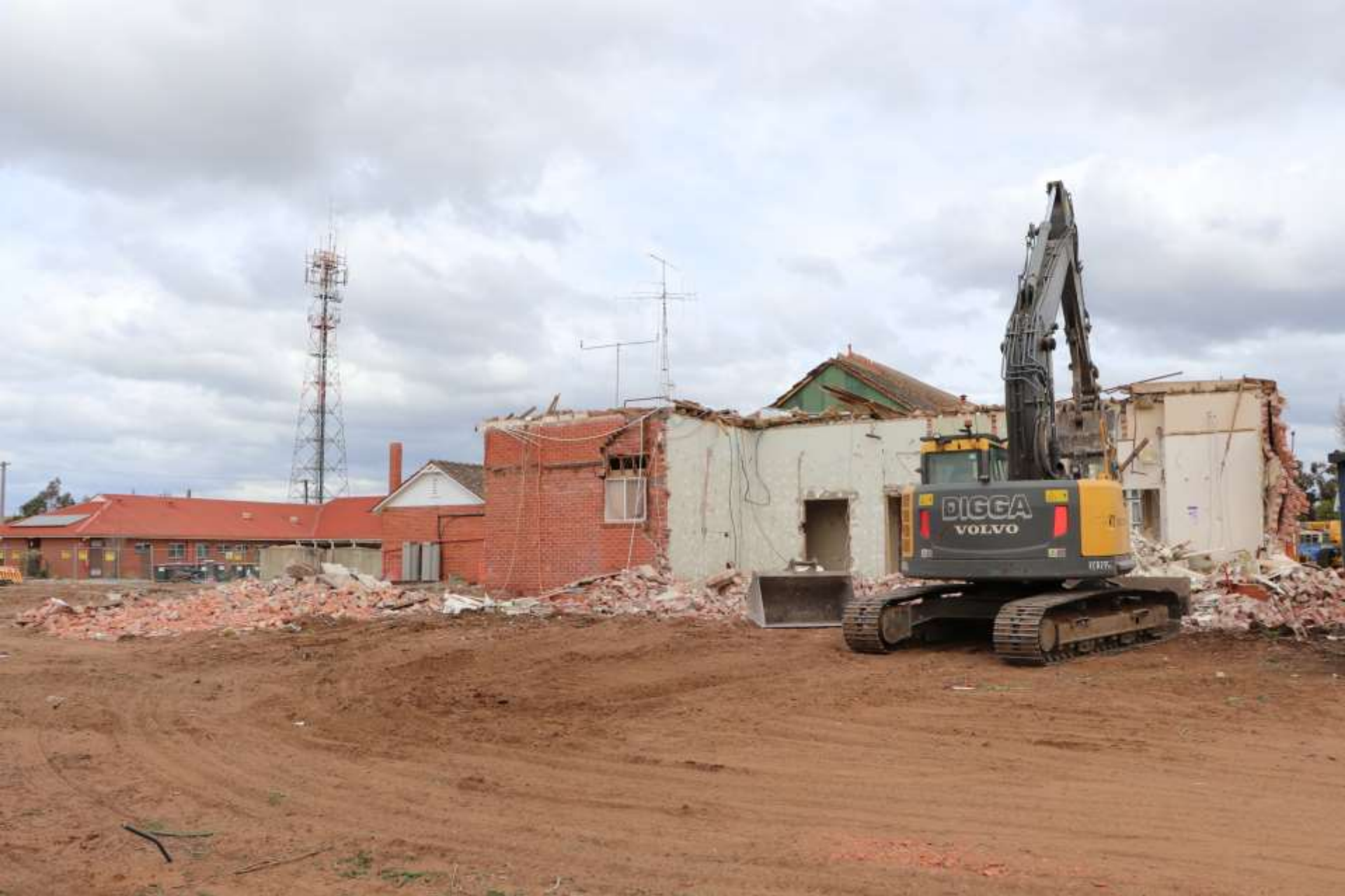
EWHS Birchip Campus – Hospital Demolition
