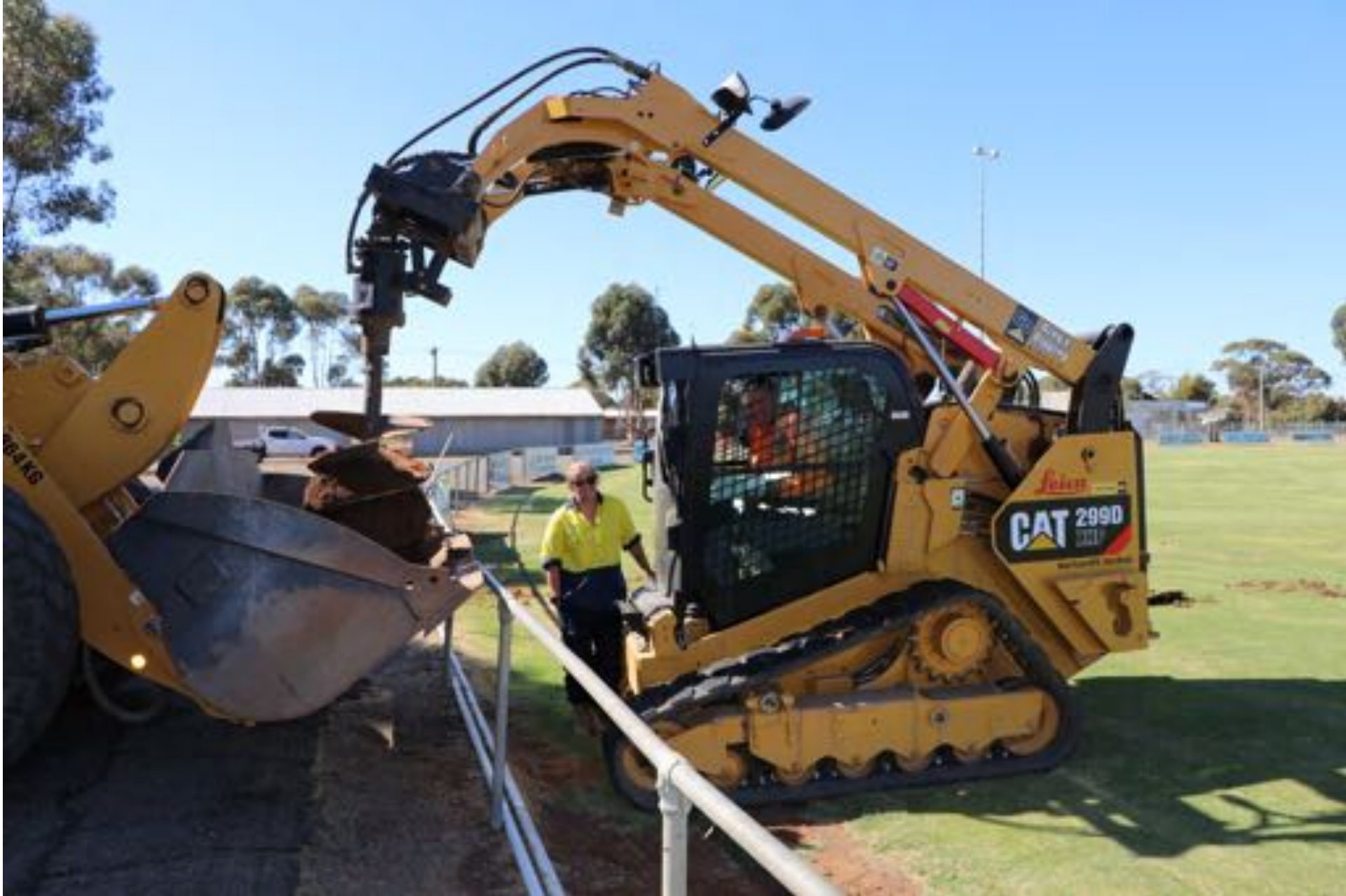
Greg Rymer digging holes for the new goal posts
