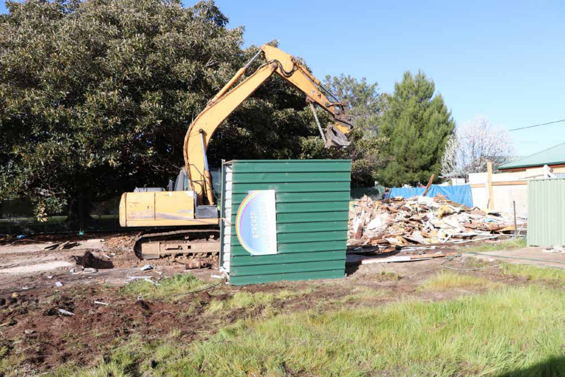
Birchip Kindergarten demolition
